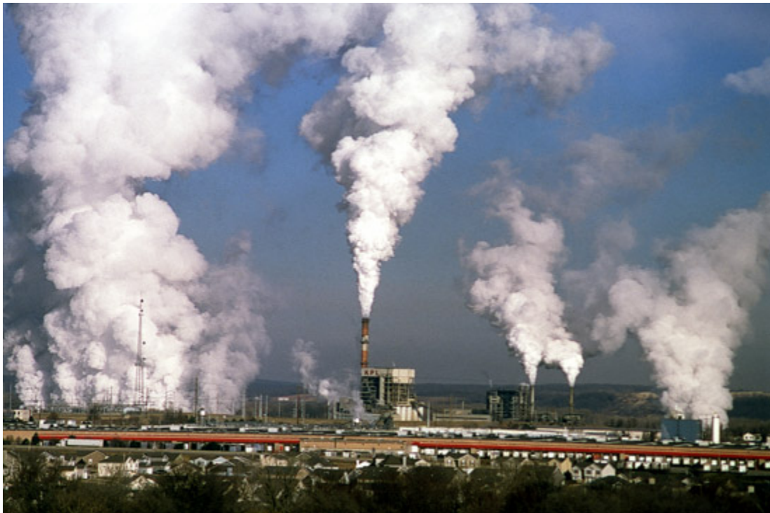
Kansas coal-fired electric plant on a cold winter's day Westar Energy's Lawrence Energy Center—Lawrence, Kansas
